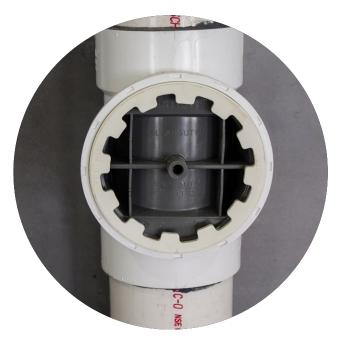
Partial tests are also easier and faster, since TESTRITE allows for partial drainage, if repairs are needed. Another plus, Kevin says: Tests can be held for the full 15 minutes required and then some, which was not always the case with inflatables, Kevin says.
